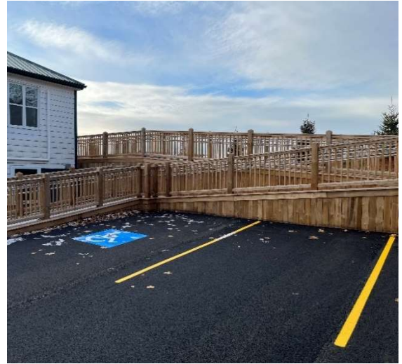
Figure 6 – Main Parking Lot
