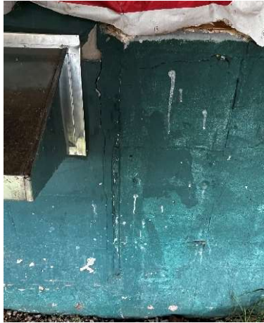
Figure 9 – Minor Cracks
