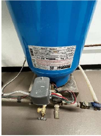
Figure 17 – Expansion Tank
