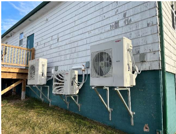
Figure 19 – Heat Pumps
