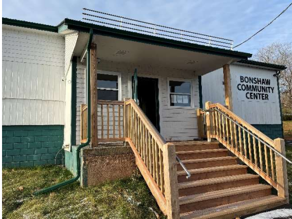
Figure 13 – Front Steps to Front Door
