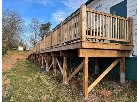
Figure 14 – Accessible Ramp to Back Door
