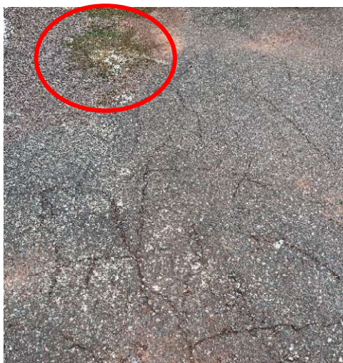
Figure 5 – Main Parking Lot (East Side)
