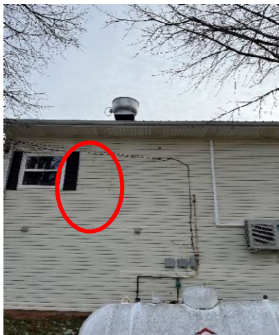
Figure 3 – Exterior of Siding at Kitchen
