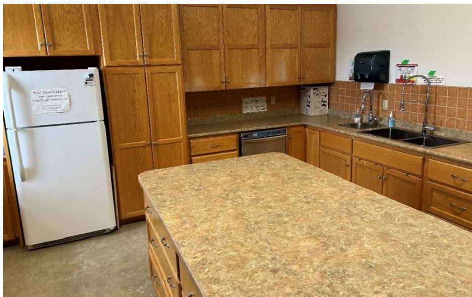
Figure 30 - Kitchen with Residential Fridge and Commercial Dish Washer
