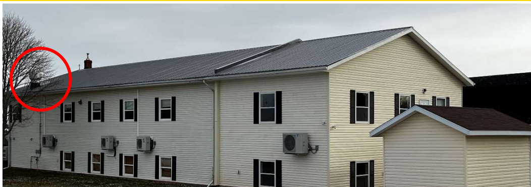
Figure 9 - Steel Roof on Original Building and Addition
