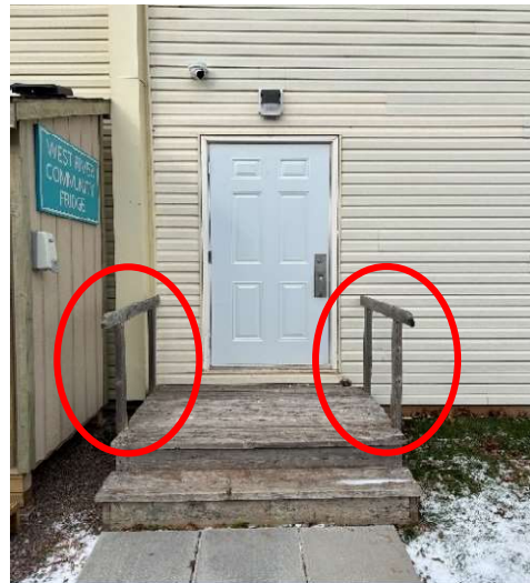
Figure 11 – Side Entrance to Elevator – Hand Rails and Steps
