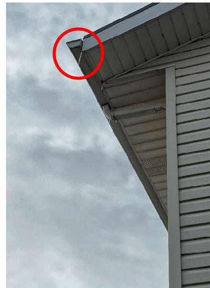
Figure 2 – Fascia Separating
