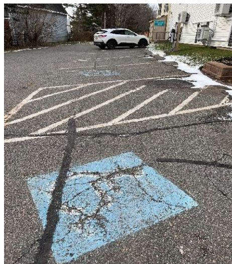
Figure 6 – Main Parking Lot (East Side)
