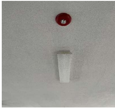
Figure 24- Fluorescent ceiling lights.
