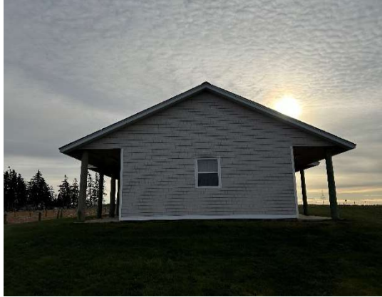
Figure 6 – Original Windows in Both Buildings
