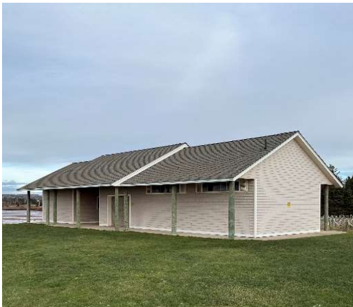
Figure 1 – Rear Exterior of Large Building
