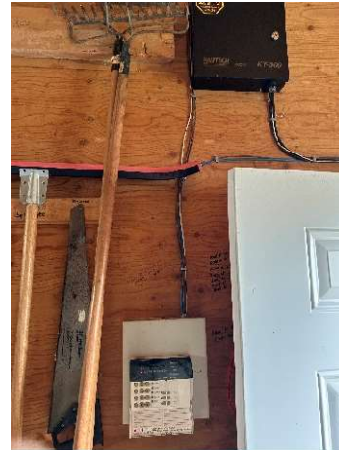
Figure 16 – Storage area interior walls.
