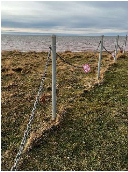
Figure 8 – Cliff Perimeter Metal Fencing
