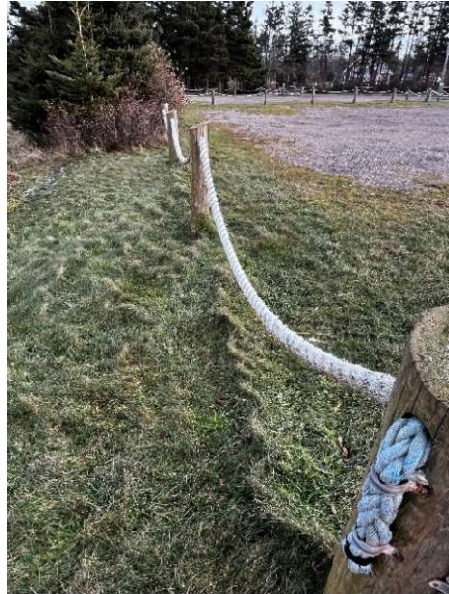
Figure 9 – Parking Perimeter Rope Fencing
