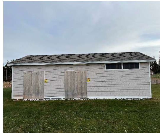
Figure 2 – Rear Exterior of Small Building
