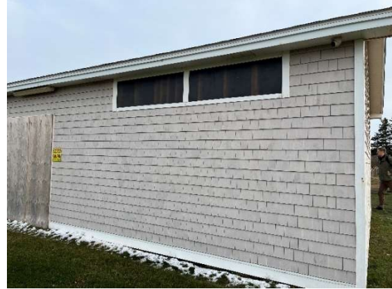
Figure 7 – Original Windows in Both Buildings
