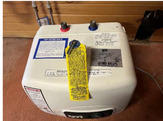
Figure 13 – Compact water heater
