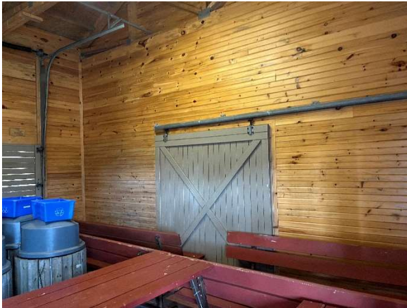
Figure 15 – Interior walls in publicly accessible areas.
